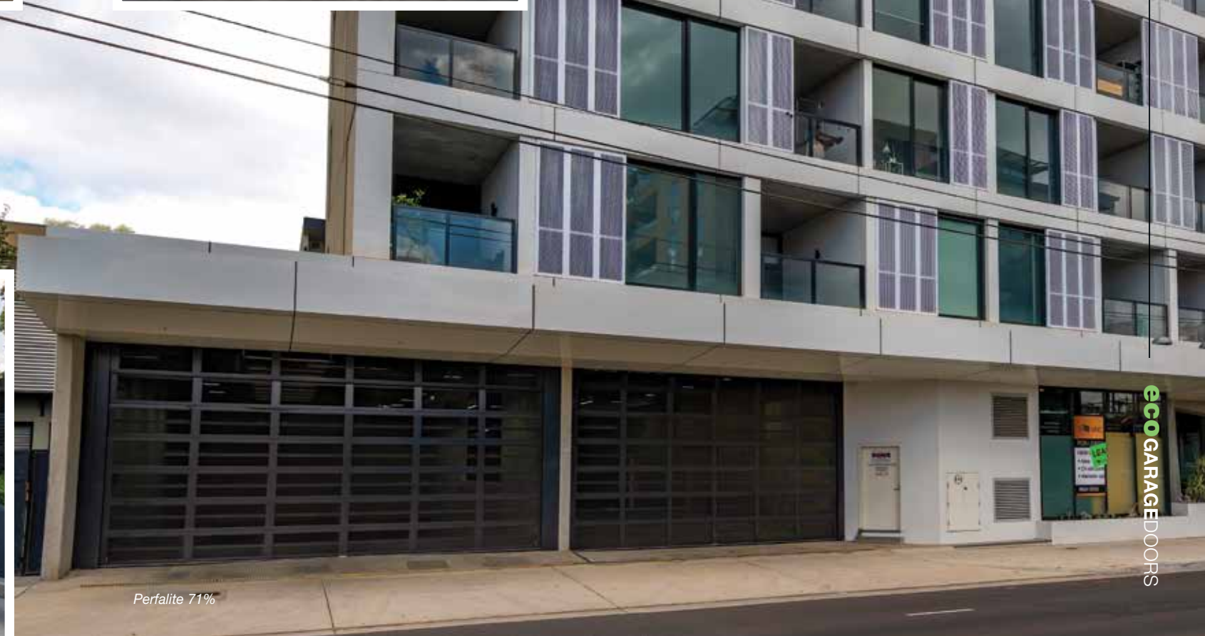
50x50 RHS vertical aluminum batten
